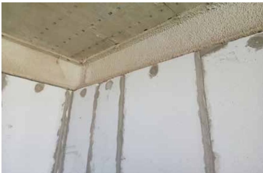
勾头螺栓法安装内隔墙
